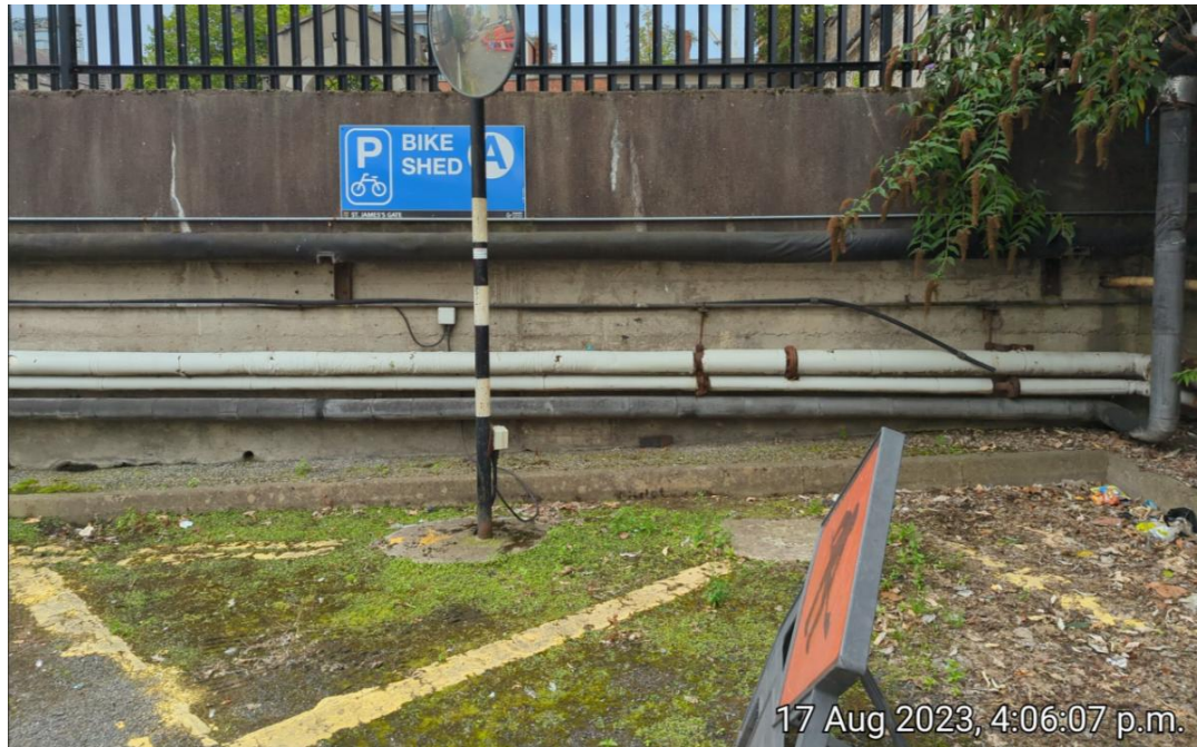
Figure 4-10: Car park boundary wall to be temporary removed
