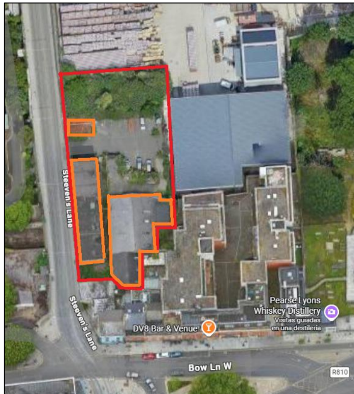
Figure 4-7: Existing Buildings to be demolished (in orange) within the proposed substation location
