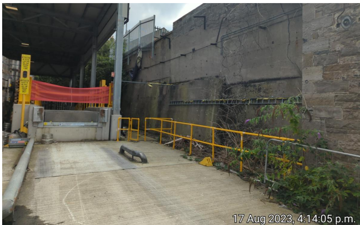
Figure 4-8: Existing Retaining Wall to the East
