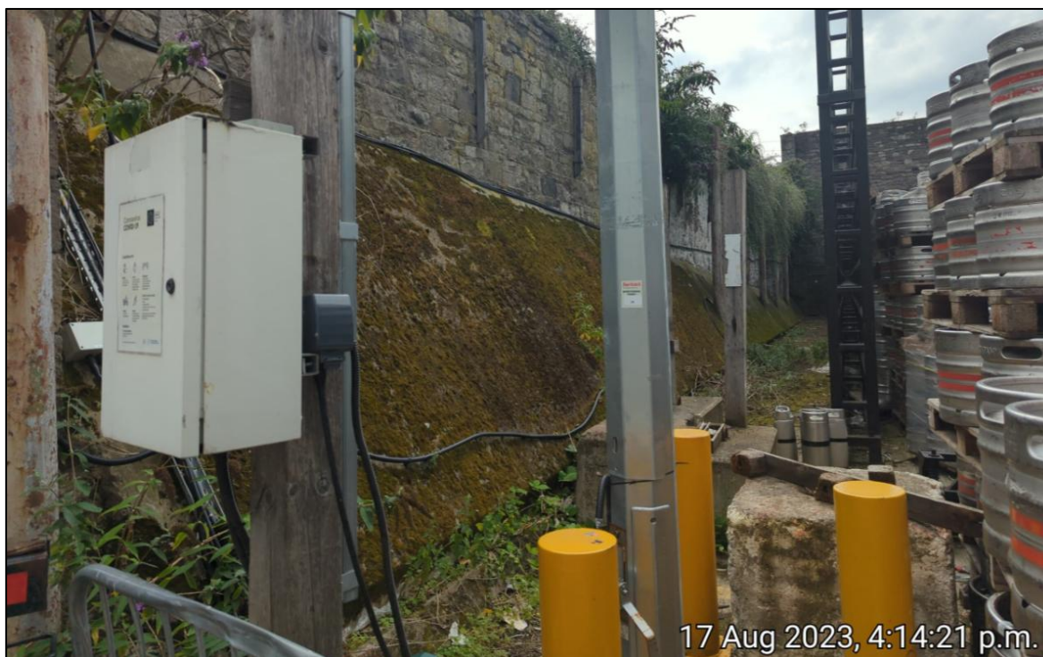
Figure 4-9: Existing Retaining Wall to the North
